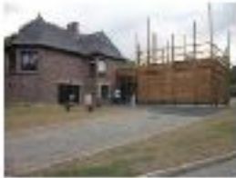
Exterior view of the building
